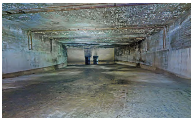
Northern section of Tiergarten tunnel, site of the WWII factory. Channels in ceiling were for street lighting and signage. Photo Clive Penfold
